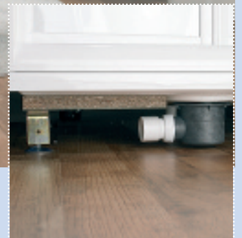
Detail showing adjustable feet and waste
